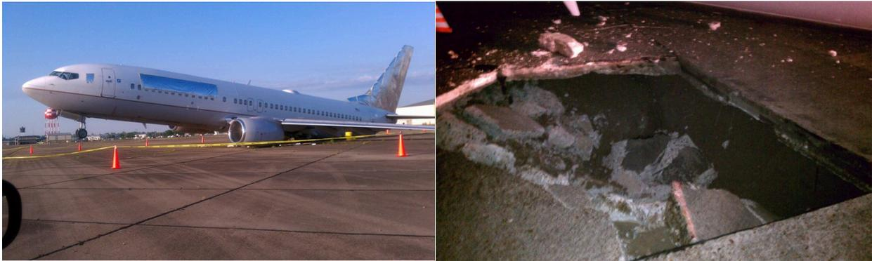
Geologists speculated that subsurface processes, associated with the flooding of the nearby Mississippi River the previous spring, caused voids to form under the concrete.
